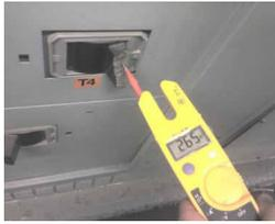
Although thermography is a non-contact test, preparing for an infrared inspection of electrical equipment often requires manual preparation of switchgear components. Unwary thermographers and their assistants can be injured by making contact with cabinets or component surfaces that have become accidentally or
