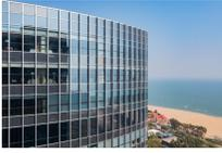
Glass curtain walls are a common feature found on modern commercial buildings. Opaque glass panels called spandrels are used to cover materials or prevent construction elements from being viewed from the exterior of the building. Examples of such areas include areas between floors, hung ceiling areas, knee-wall areas below vision lights, and sometimes even columns or partitions.
