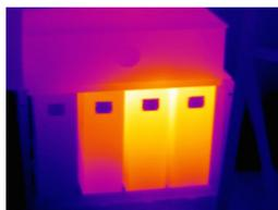
Capacitors are wound devices that are electrically connected between potential and ground. Capacitors used for power factor correction are generally encased in painted, rectangular steel canisters and often have two equal sized bushings for electrical connections. In a three phase circuit, there may be several capacitors connected to each phase.
